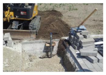
Backfill and ensure riser is set correctly. Conclusions of the Enbridge Gas exercise
