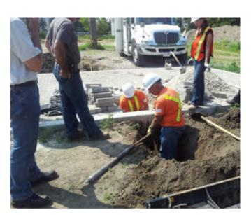
Torpedo and hose are pulled up and out of the pit.
