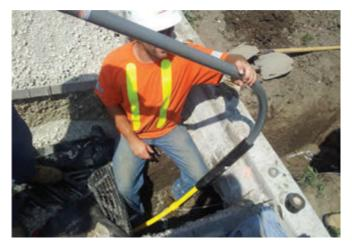
Riser is attached and pulled through.
