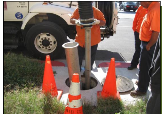
Insertion of vacuum hose into separation chamber.
