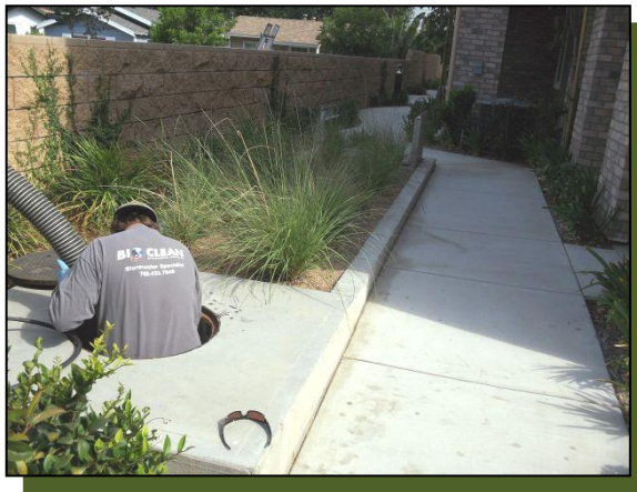
Vacuuming out of media filters.
