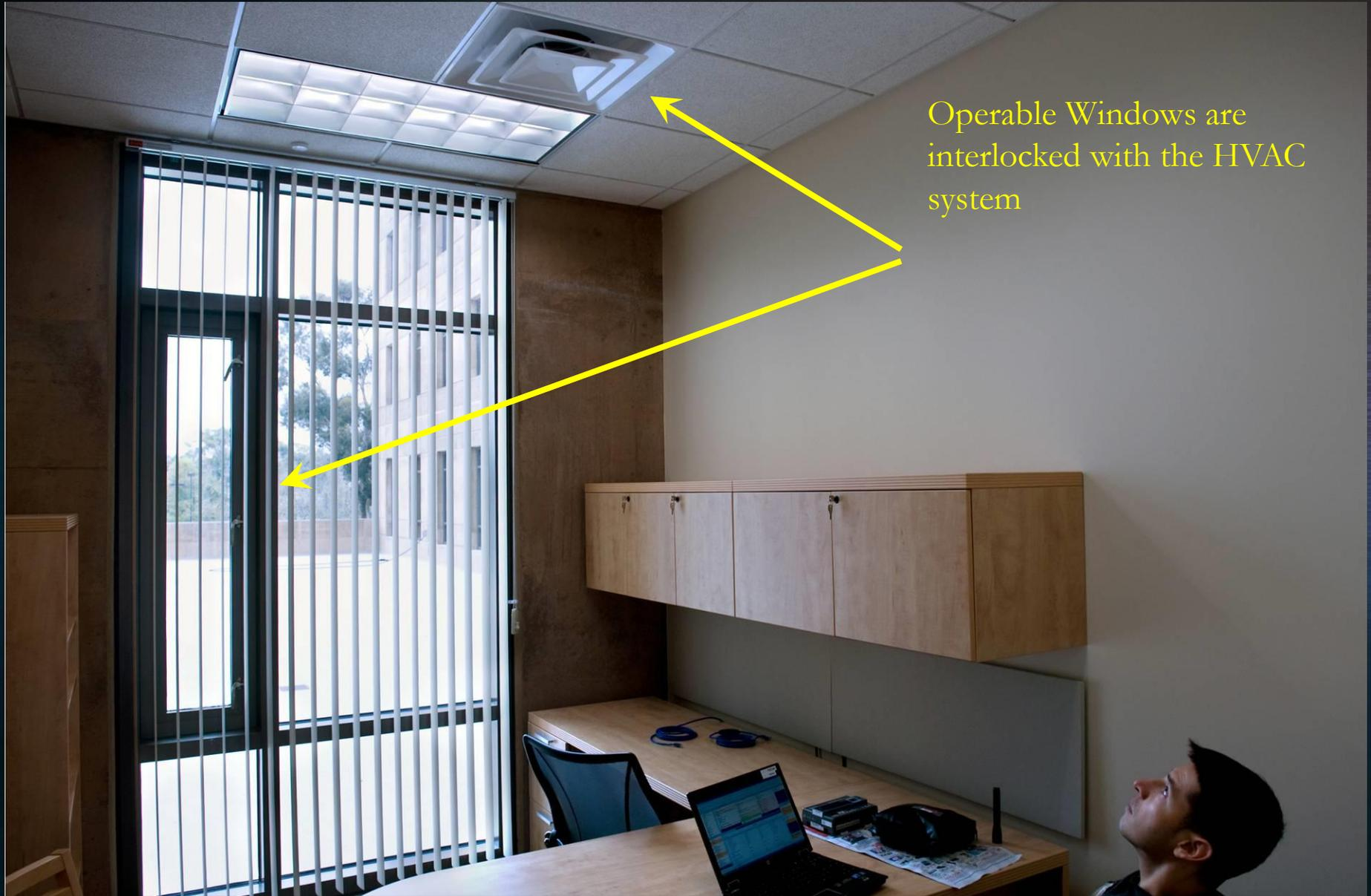
Operable Windows are interlocked with the HVAC system
