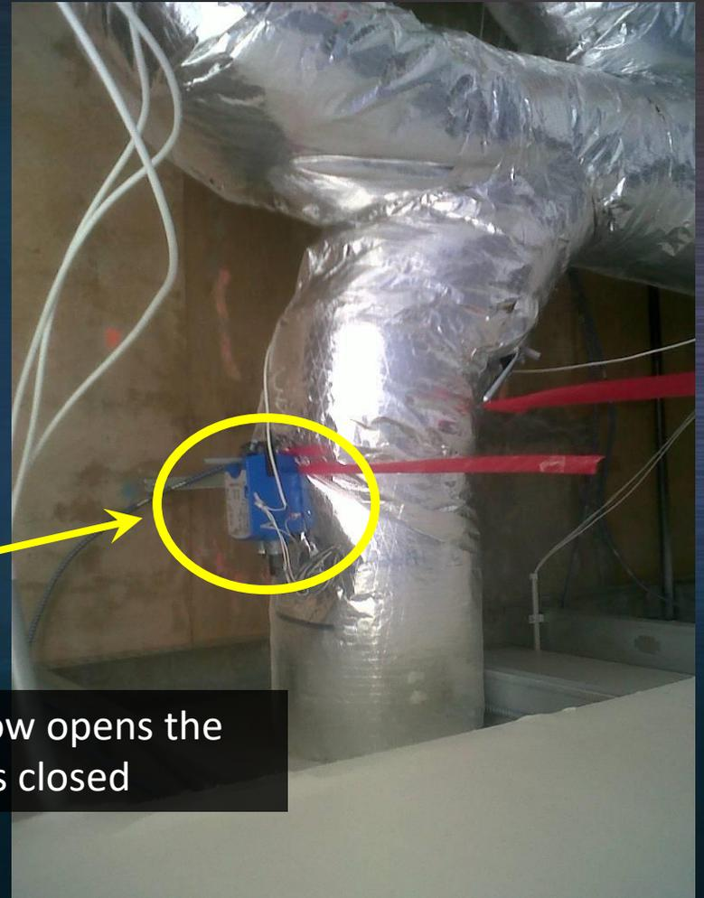
When the window opens the supply diffuser is closed
